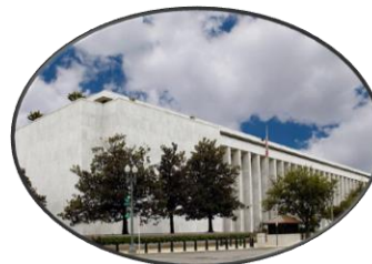
James Madison Memorial Building
